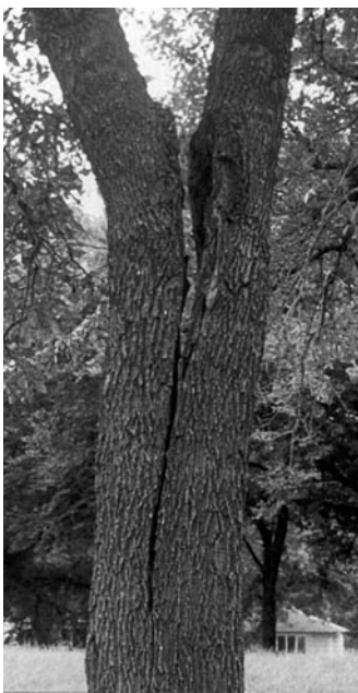
This weak branch union has developed a crack, creating a highly hazardous situation.
