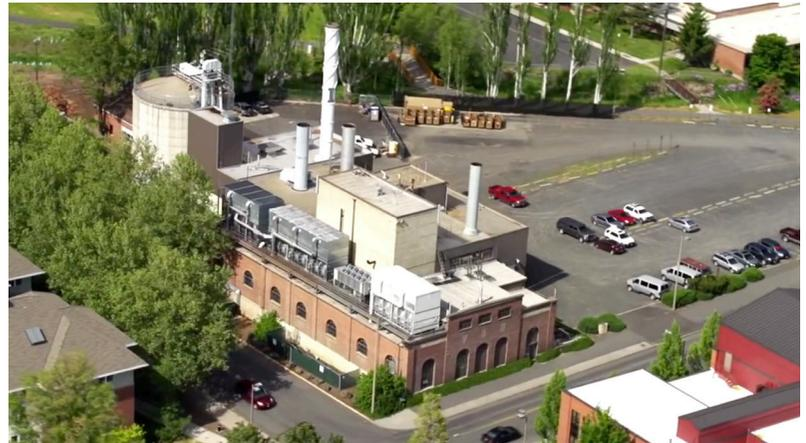
Nestled within the campus of the University of Idaho, steam for hot water in the dorms and heat to warm all buildings in the campus core area come from this wood-burning boiler plant.
