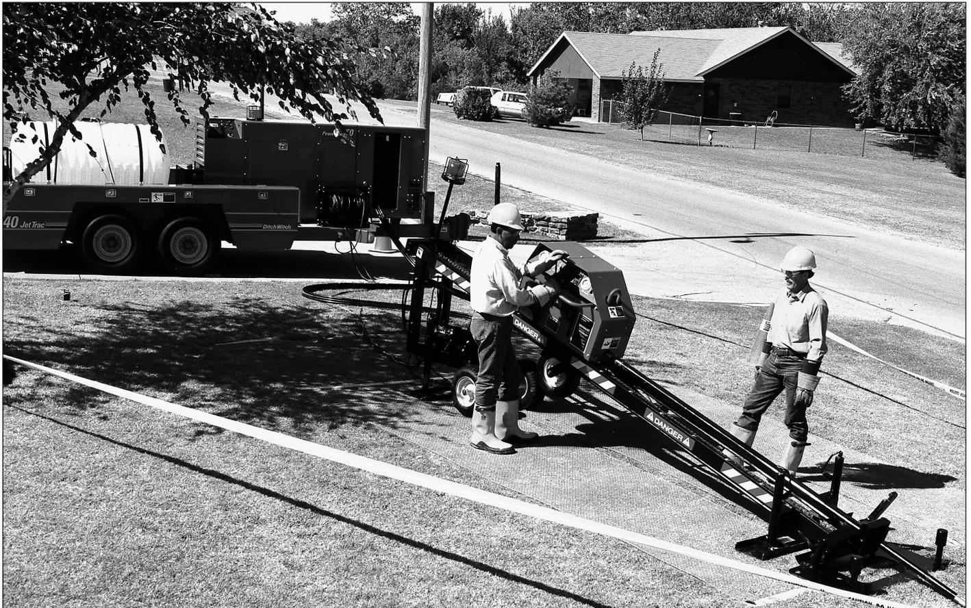
*Modern equipment is able to tunnel safely beneath the roots of a tree. It is widely available and used increasingly by utilities and construction companies.*
