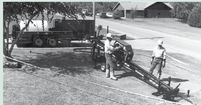
Modern boring equipment enables utility companies to tunnel safely below a tree's critical root zone.
